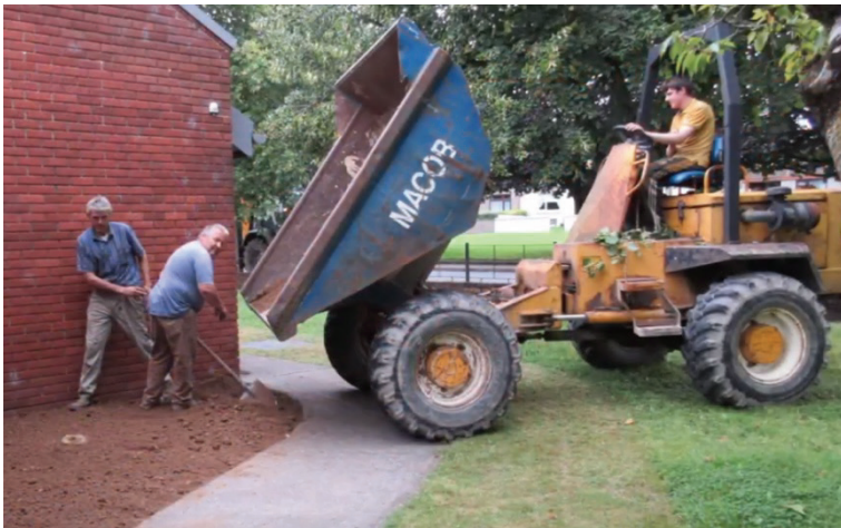
After calculating how much top soil was needed, the soil was delivered and spread across the site.
